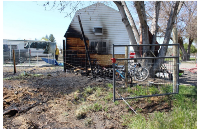
An outdoor burn was reported extinguished after water was applied.
